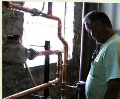
Plumber George Jonas puts the finishing touches on new copper pipes.
