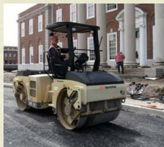
A new layer of asphalt is smoothed down around the Courthouse.
